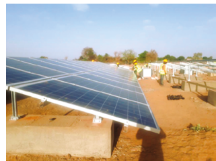
Installation of photovoltaic panels for an electricity supply project in Burkina Faso.
