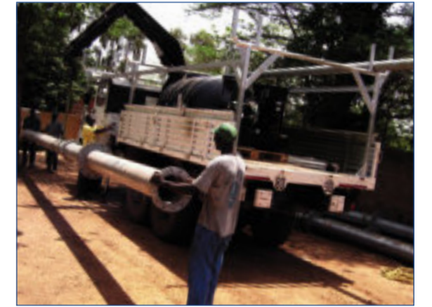
Unloading of a mast-mounted tank
